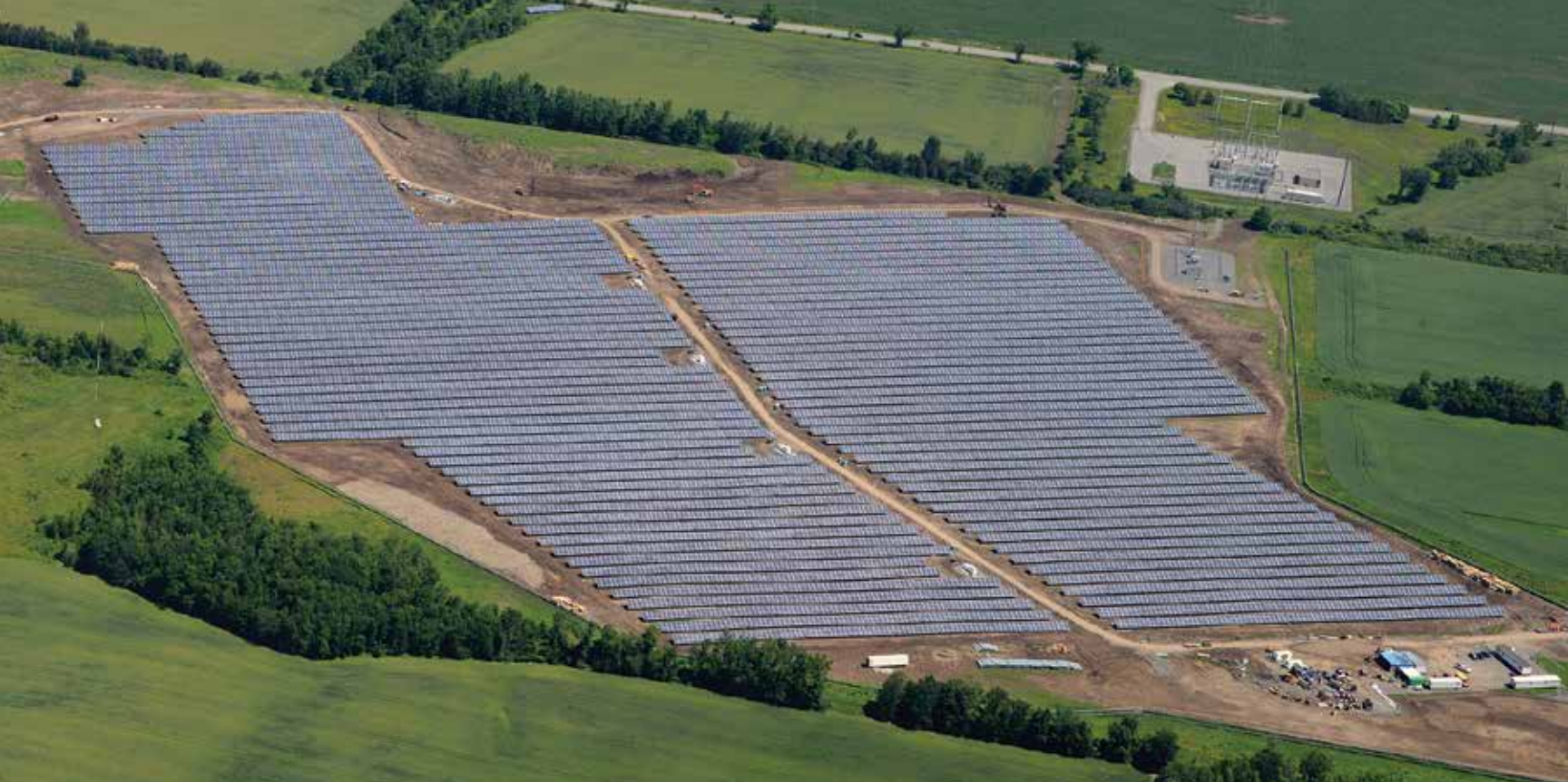
Sunny Shores Green Energy Solar Park, 14 MW
